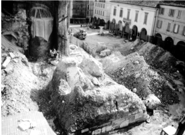
Fig. 3. The Bell Tower of Pavia after collapse
