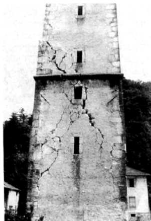
Fig. 22. Crack pattern of a bell-tower and interpretation of the damage mechanism [Doglioni, 1994].
