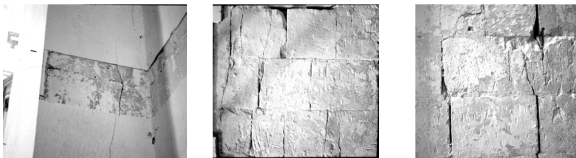
Fig. 58. The appearance of a crack on the plaster and underneath it [Binda, 2001]
