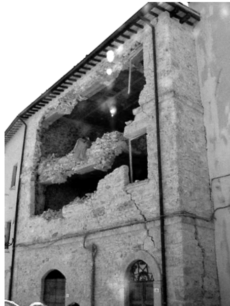
Fig. 1. Damages after Umbria earthquake to a building repaired by introduction of concrete tie beams.
